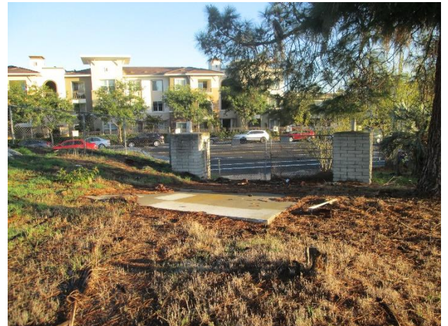
12. Concrete slab and entrance gate in the northeast corner of the Site.
