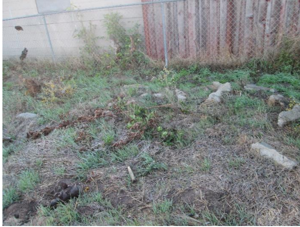
14. Concrete debris in the eastern portion of the Site.
