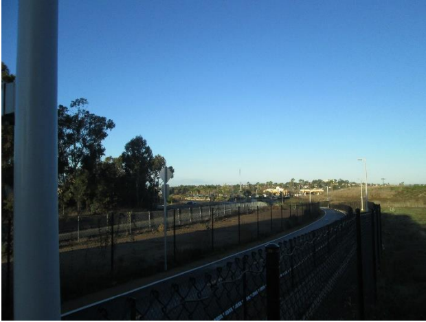
19. Southern adjacent railroad tracks.
