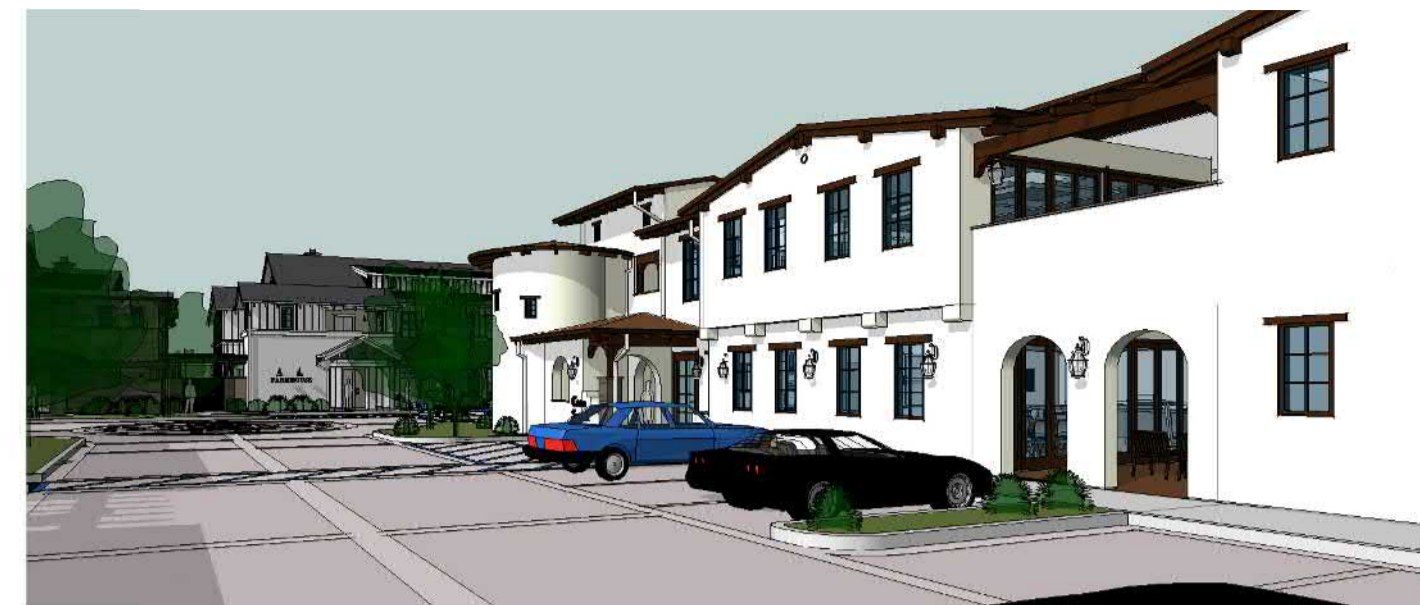
Arrival Drive & Casa Santa Barbara Entry
