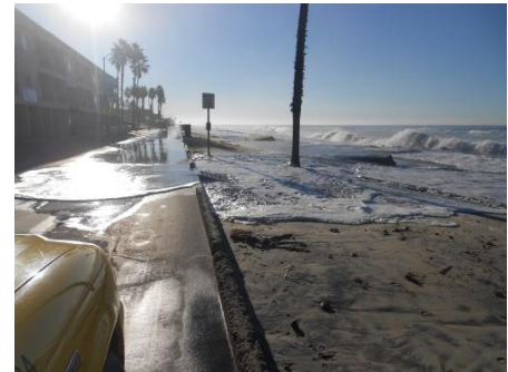
Coastal flooding on the Strand
