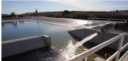
Oceanside’s reclaimed water is kept in a reservoir before it is pumped to the Oceanside Municipal Golf Course or a bird sanctuary
