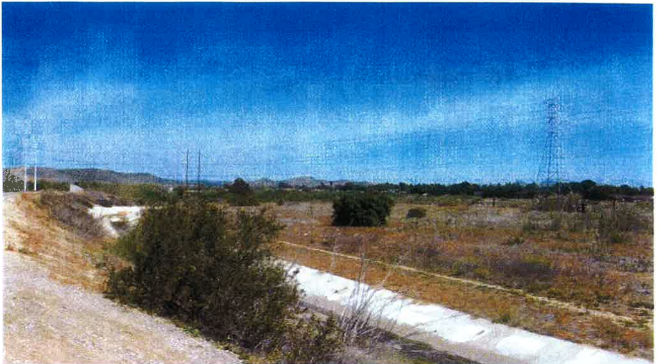
Looking northeast along river levy of SDG&E transmission line east of desalination plant.
