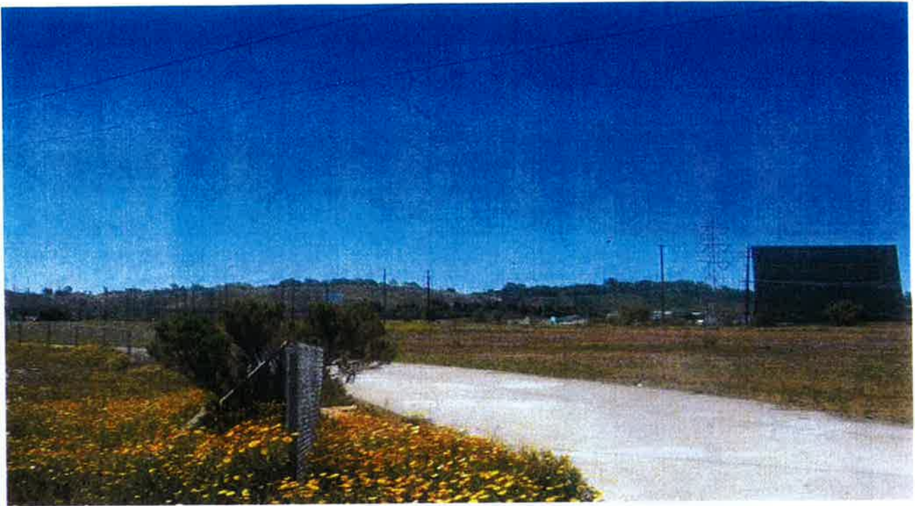
SDG&E transmission line along the eastern boundary of Pavilions project site – north end. The concrete “road” covers an existing storm drain paralleling the transmission corridor.
