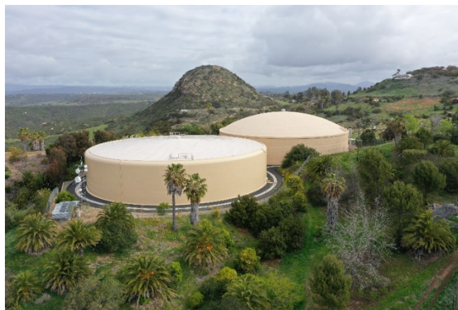
Rehabilitation of the Morro Hills No. 1 & No. 2 Reservoirs
