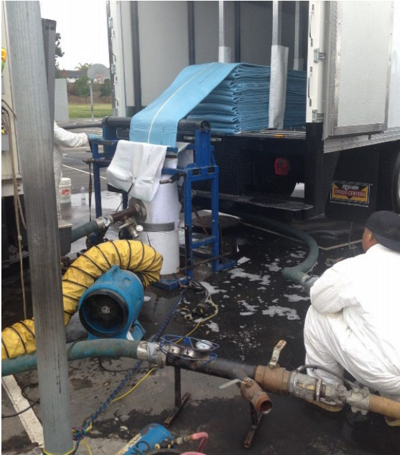
Installing Cured-In-Place-Pipe (CIPP) slip lining to rehabilitate the City's pipelines and protect against leakages and water quality contamination.
