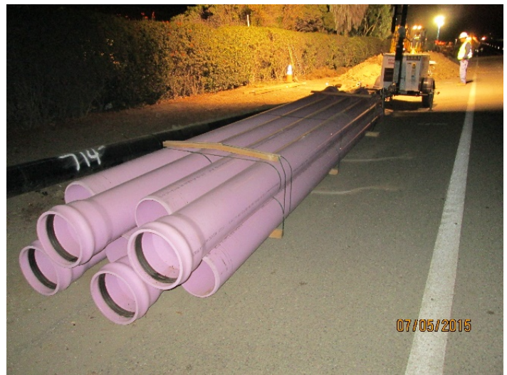
Installation of recycled water pipelines constructed as part of the Recycled Water Conversion and Pipelines Project
